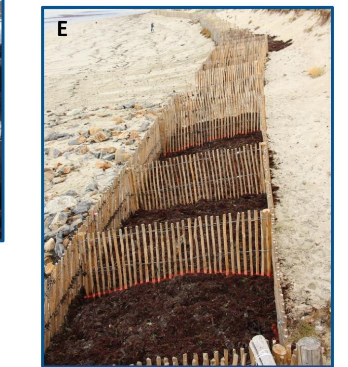
Series of photos showing: (A) initial state of the beach, (B) AlgoBox, (C) AlgoBox implementation, (D & E) AlgoBox filling by red algae.
